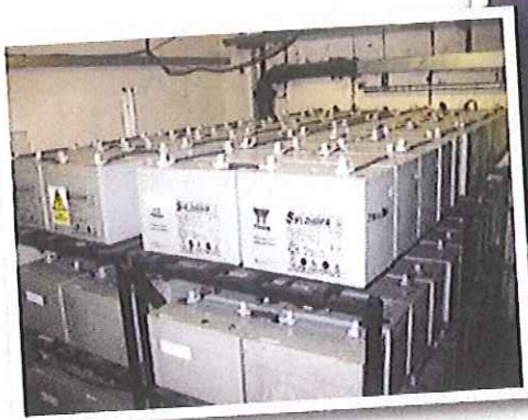
The Installed PowerWAVE9000DPA Modular UPS System and battery banks supporting all emergency lighting for both front and rear of house
