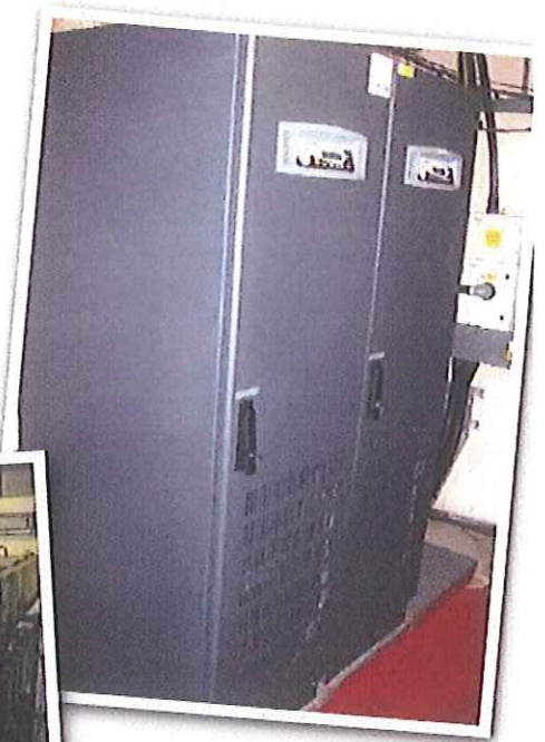
The Installed PowerWAVE9000DPA Modular UPS System and battery banks supporting all emergency lighting for both front and rear of house
